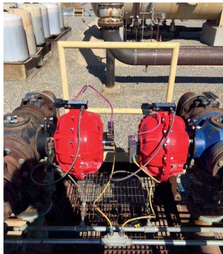
Figure 2: New generation fail-safe actuator without the use of springs for better durability, safety, efficiency and cost. New generation actuators fit where rack & pinions can not.
